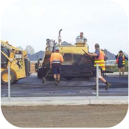
The court under construction at South Colac
