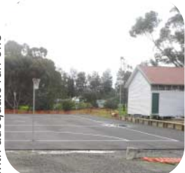
After: new asphalt playing surface with adequate run offs
